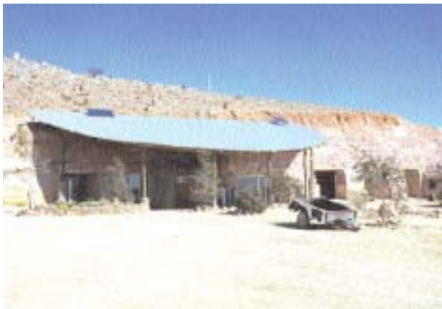
In the Australian town of Coober Pedy, many homes are built into the desert rock, which keeps interiors cool during the day and warm during the evenings.
